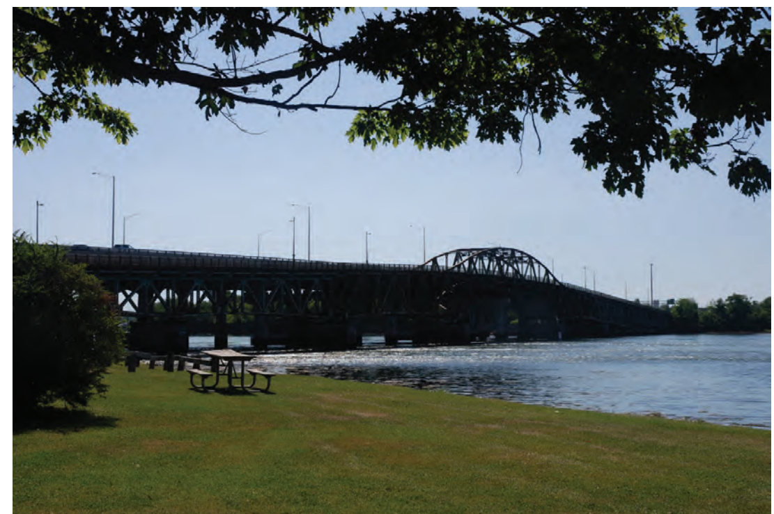
8. Looking to south toward GSB from west side of Hilton Park. July 12, 2018.
