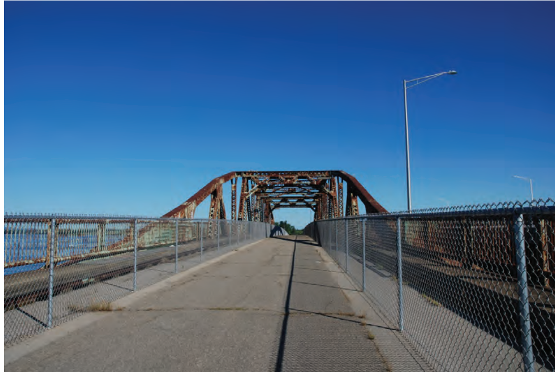
5. Pedestrian view north on the GSB deck toward Dover. July 12, 2018.
